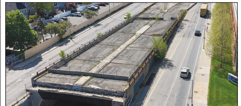
The aerial view of the Rutherford Avenue tunnel as it currently exists.
