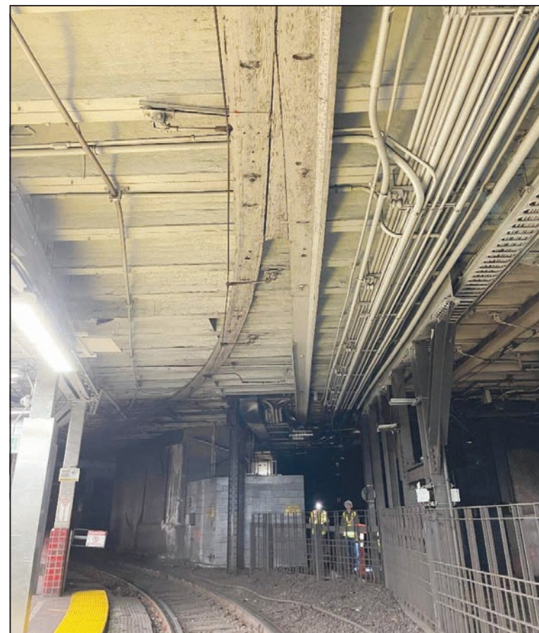
The wooden overhead catenary trough – seen here at Park Street – dates back to the late 1890s and will be replaced with a modern, more durable, metal trough.
