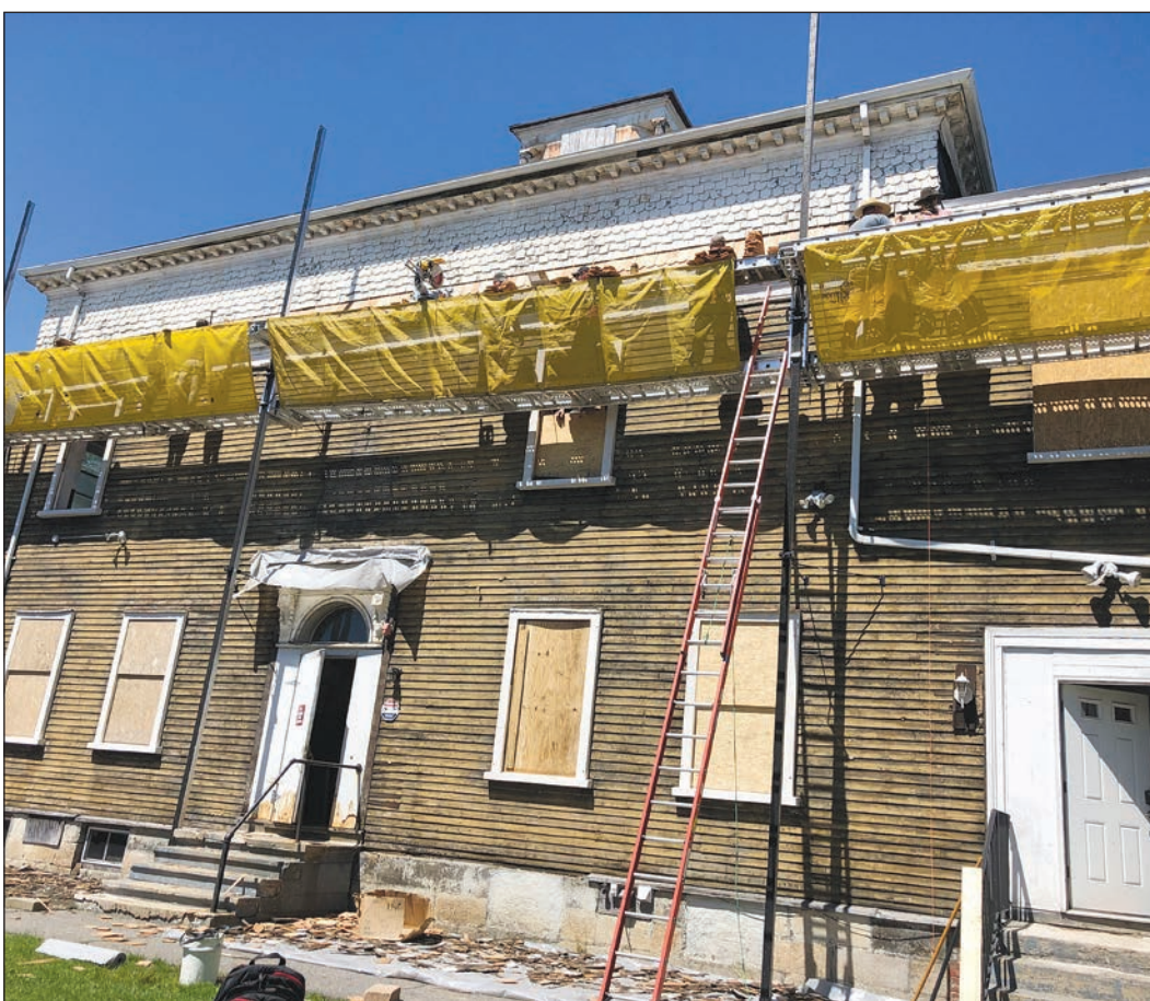
Shingles have been removed and the original clapboard is exposed.
