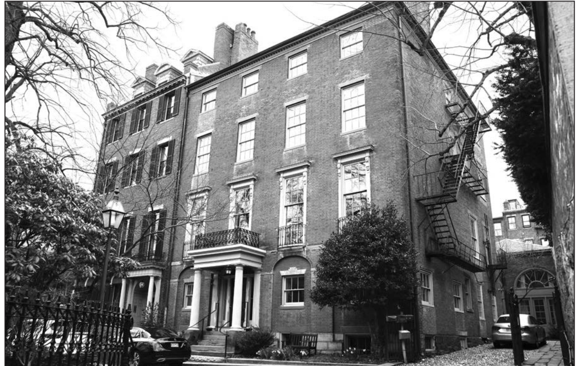
The house on 87 Mount Vernon Street.
